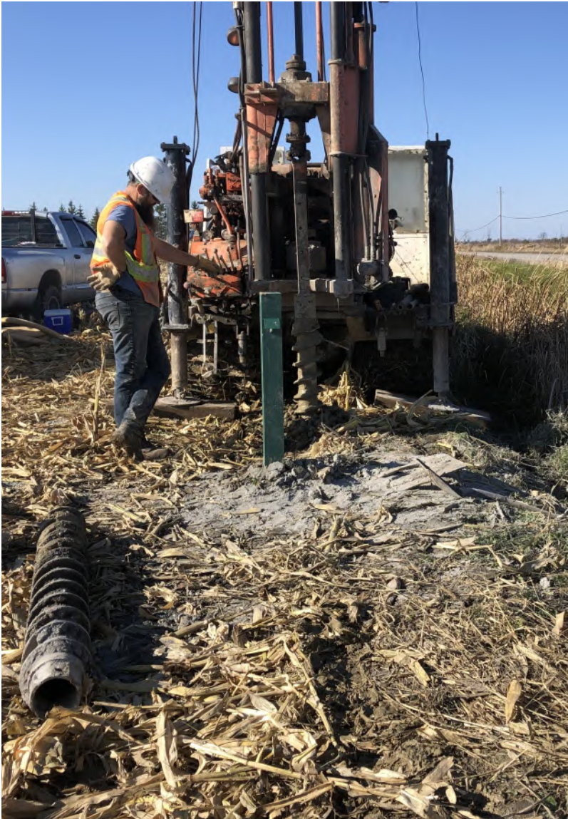
Photo 30: view of MW201 and MW202 installation.
