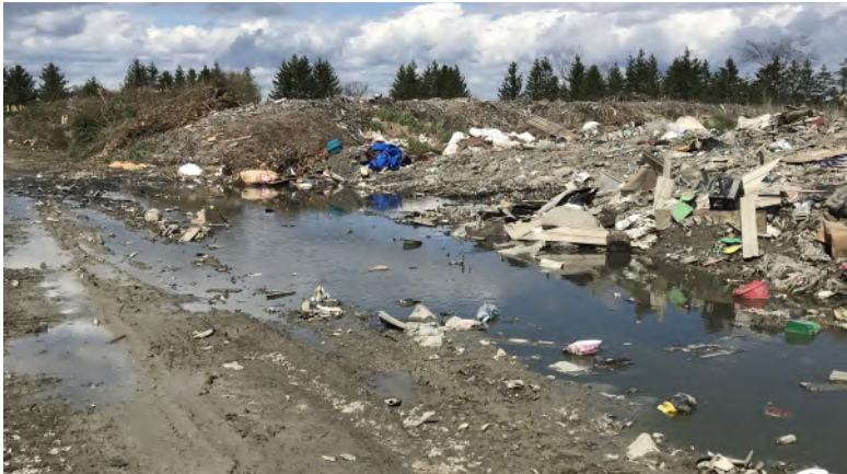
Photo 28: view of ponded water observed on site
