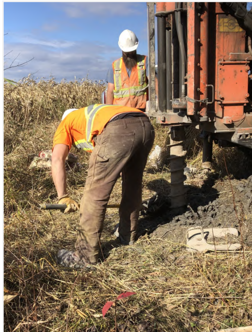
Photo 31: view of MW203 installation.
