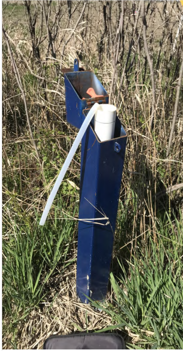
Photo 24: view of monitoring well MW105.
