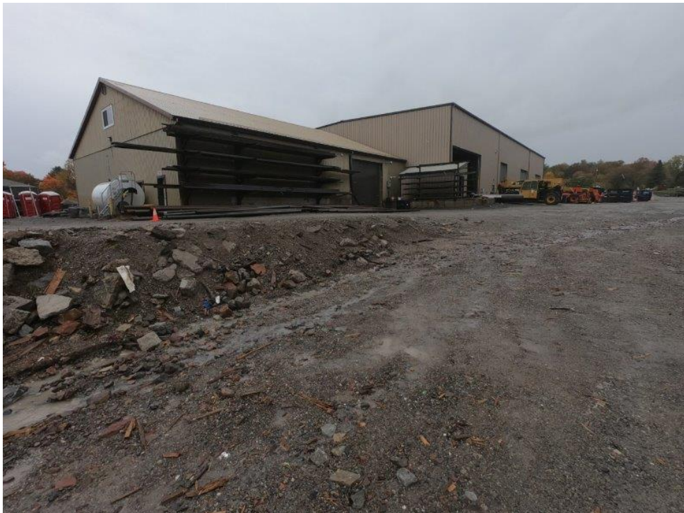
Photo A10: Upland of boat ramp, existing central building (2022)
