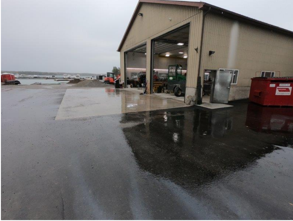
Photo A12: Existing large maintenance building and fabrication shop (2022)
