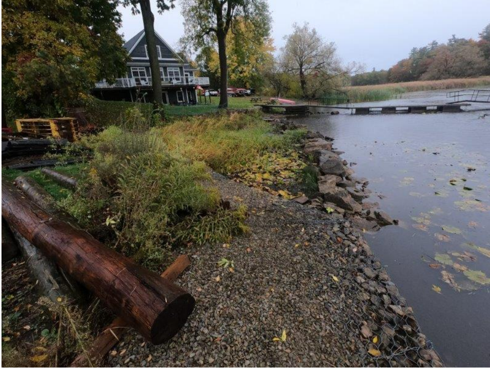
Photo A5: Looking Northeast alongshoreline, North end of gabion wall section (2022)
