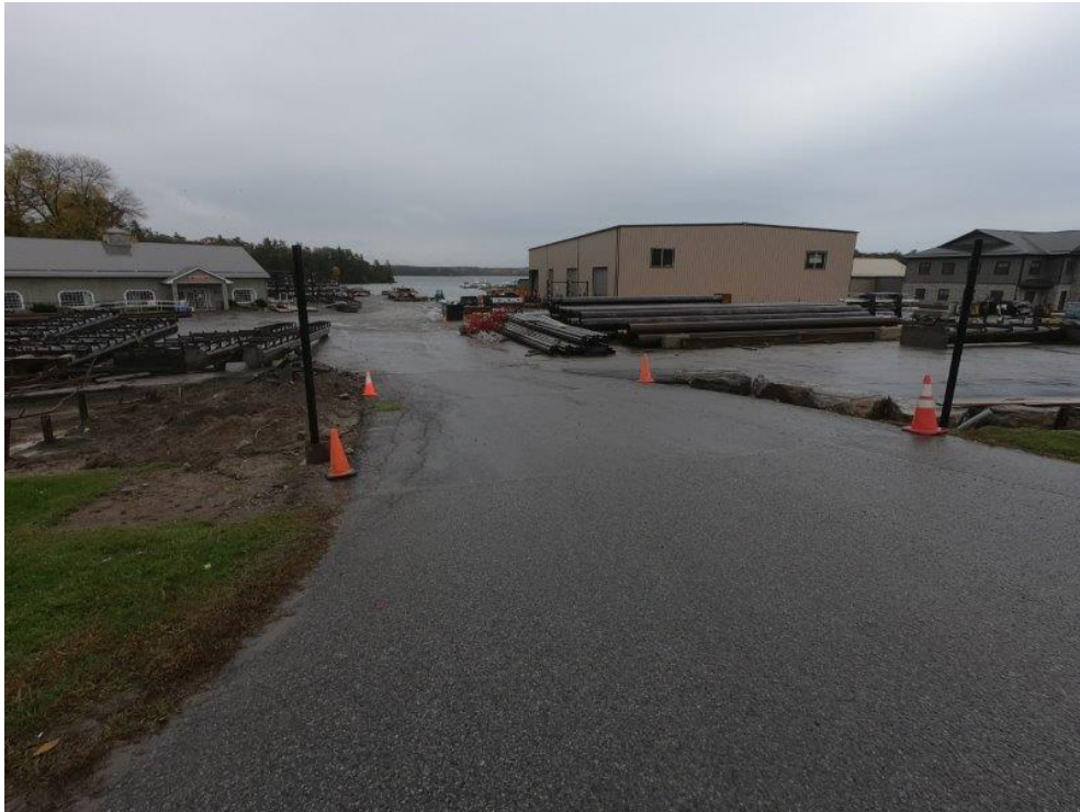
Photo A3: Looking South from Thousand Islands Parkway, eastern driveway entering property (2022)
