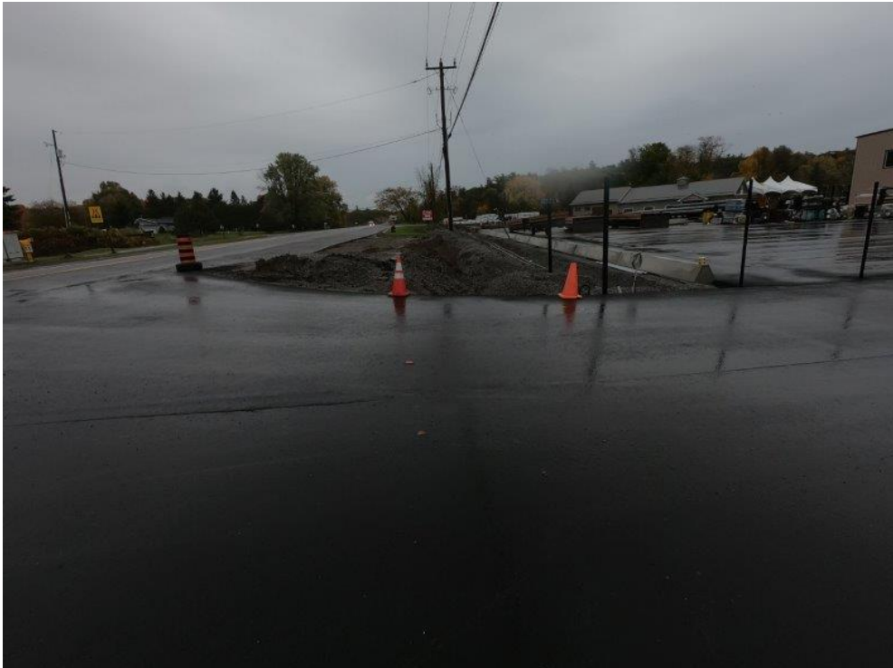
Photo A2: Looking East along Thousand Islands Parkway, western driveway entering property (2022)
