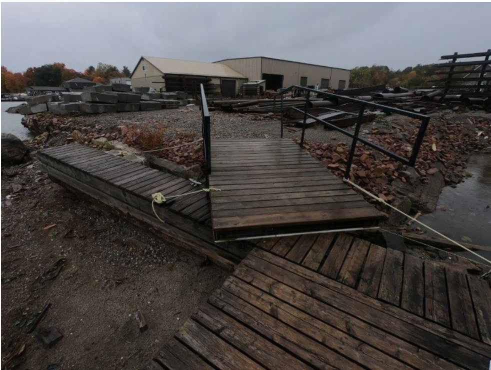
Photo A8: Rip-Rap Revetment (2022)
