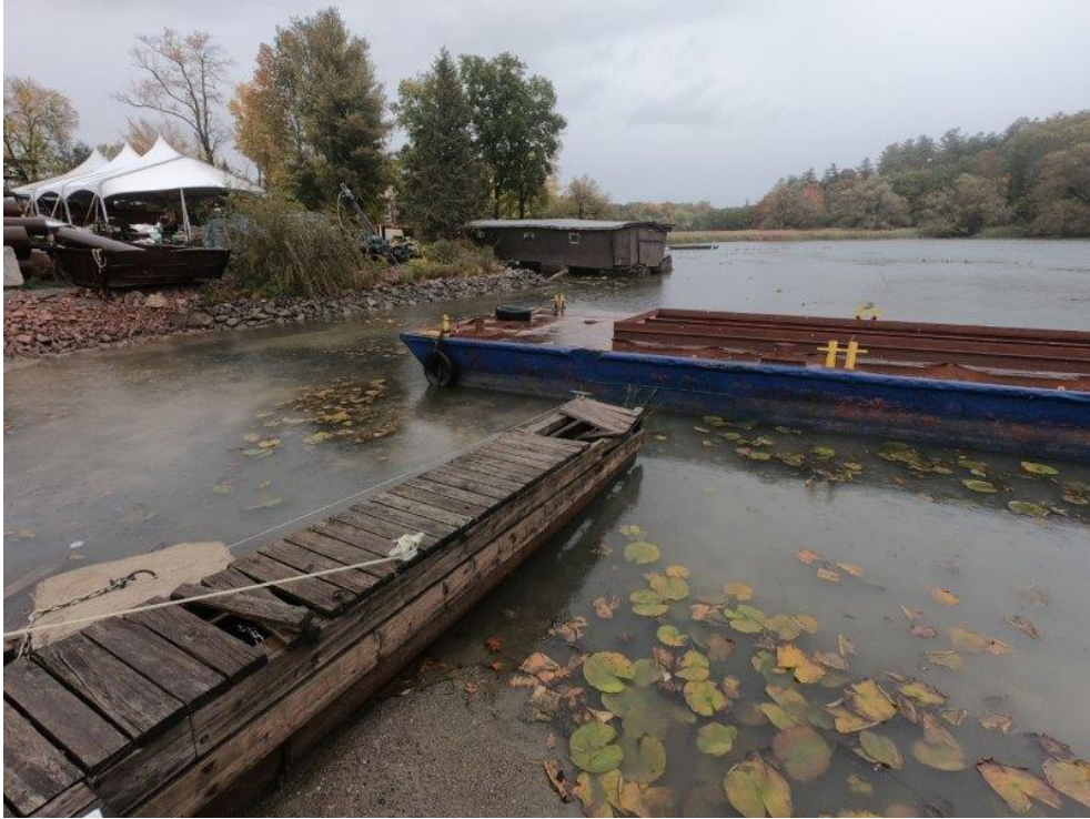
Photo A7: Looking Northeast along the shoreline towards the boathouse, at rip-rap revetment (2022)
